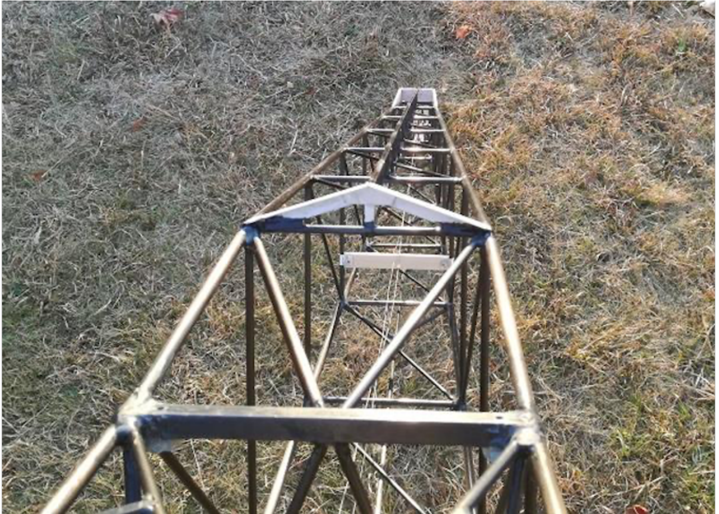
Photo 117: The completed upper overhang structure.
