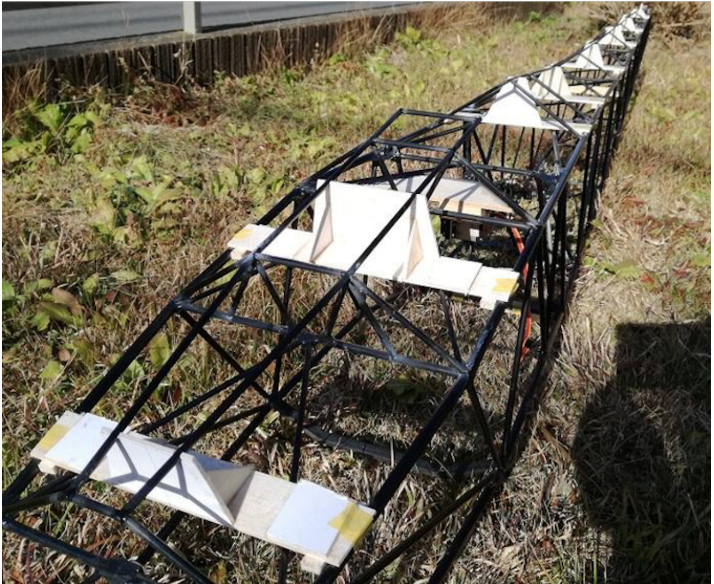
Photo 113: Assembling the lower overhang structure.
