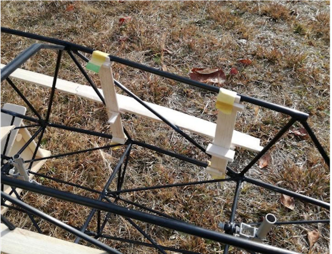
Photo 119: Installation of the side overhang using a simple positioning jig.
